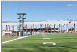
The framework of Legacy Pavilion was completed on March 15 and construction on the roof began.
