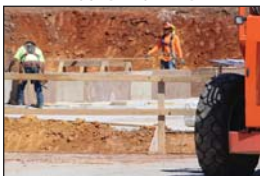
Cement was poured on October 5 for the foundation of the Football Operations Center.
